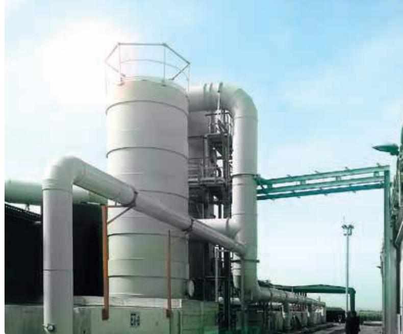
Scrubber Solutions may only be water for water-soluble substances or solutions with reagents that specifically target certain inorganic compounds to be neutralized. The design of the plant and the choice of the chemical reagent depends on the substances contained in the gas to be purified.
