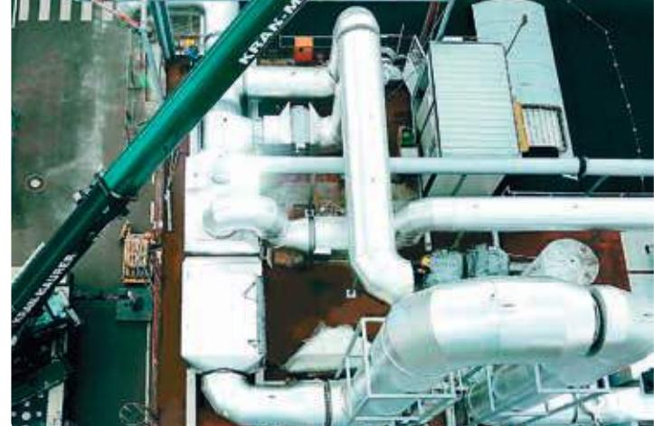
Nitrogen oxides NO<sub>x</sub> are removed by a Selective Catalytic Reduction composed of an active catalyst operating in combination with injected ammonia or urea into the process gas. This converts the nitrogen oxides (NO and NO<sub>2</sub>) to nitrogen (N<sub>2</sub>) and water (H<sub>2</sub>O). The required performance can be achieved at low temperatures, supporting the overall energy reduction program of the facility.
