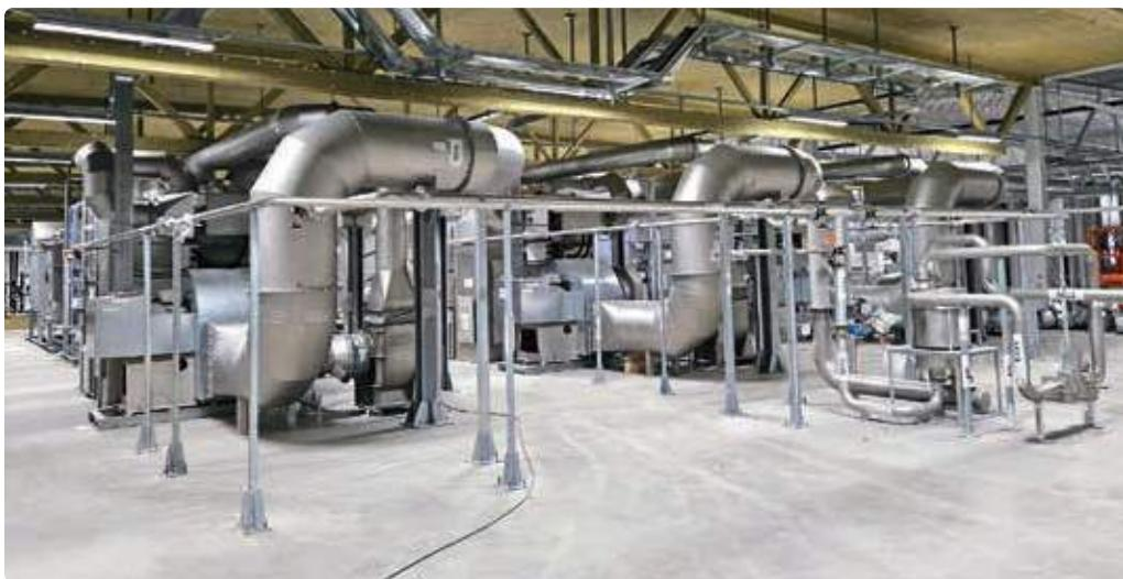
Air treatment and heat recovery systems for emissions coming from laboratory lines, pilot lines and giga-factory lines. These systems are fully integrated into production processes and guarantee maximum performance. Emissions from cathode coating are treated by condensation and adsorption processes aimed at solvent recovery, thermal recovery and compliance with regulatory limits. Coating on the anode allows for significant thermal recovery of emissions through air/air and air/water exchangers.
