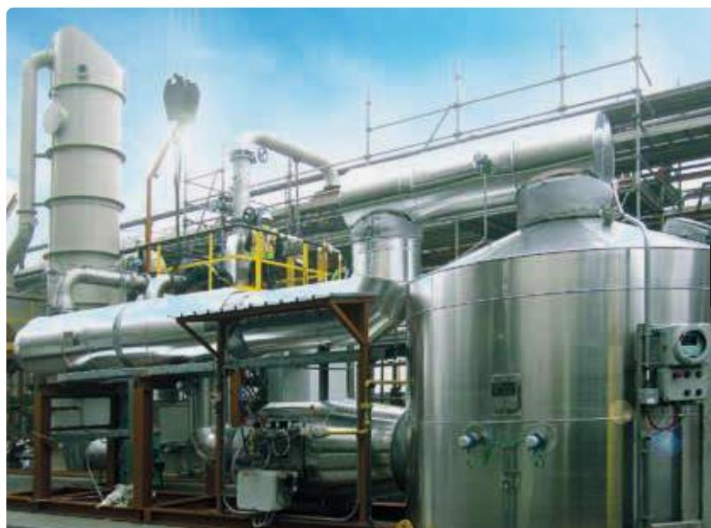
A catalyst is used to reduce the reaction temperature and therefore the energy consumption. This allows the oxidation process to be performed at lower temperatures between 300°C and 500°C, which leads to considerable energy and cost savings.
