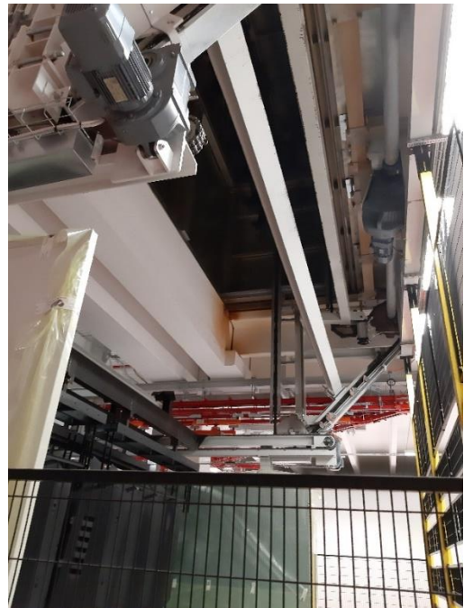
Side view of entrance to cooking oven
